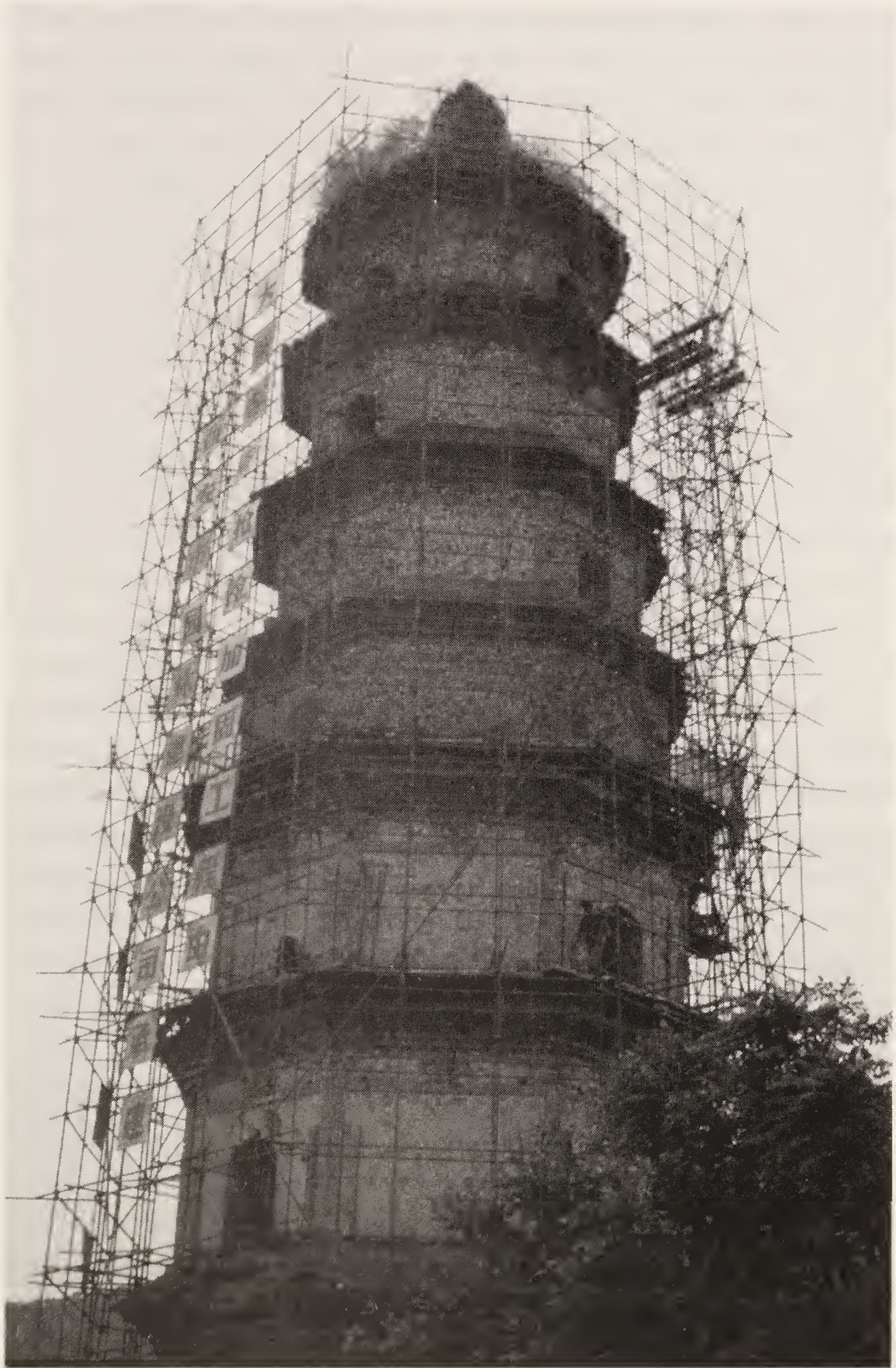
Restoration of pagoda in progress. (© Tjalling Halbertsma/CIRCA)
